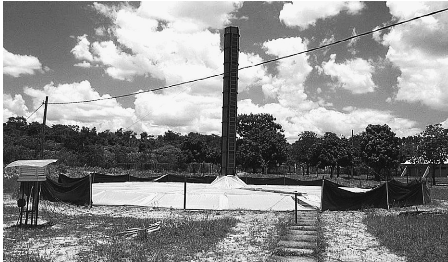
Fig. 2. Solar chimney prototype.
